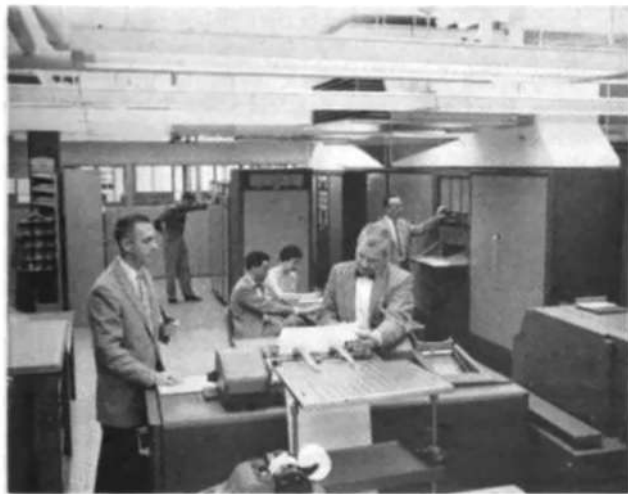
Fig. 5 – Cooling unit for a computer at General Electric, Rome, Georgia, ca. 1957. 18
